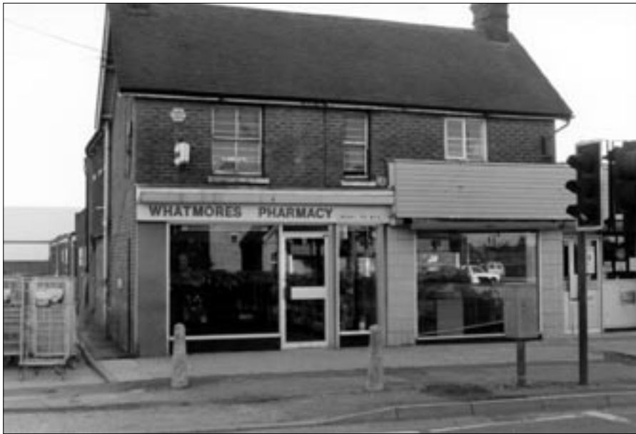
The original Blake house now heavily disguised within a modern shop front. To the rear, on the left-hand side, can be seen what is probably the new Budgens store under construction. Within days of the new store opening this front parlour shop with its many extensions was demolished.
