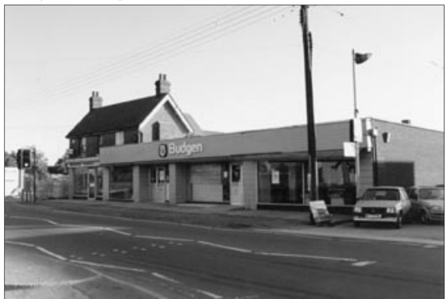
An external view of Budgen's from the 1970s-80s, with the original Blake house, now the pharmacy, still clearly visible at the left hand end.
